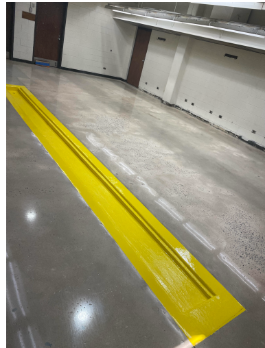
Figure 2 Concrete floor polished and floor drain painted
