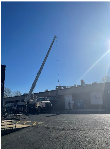
Figure 1 Crane setting new HVAC unit
